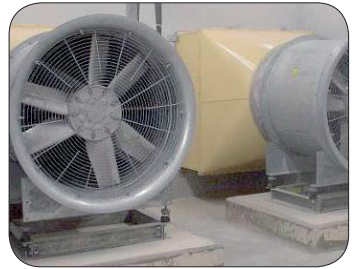
Figure 15: Example of local exhaust ventilation.
