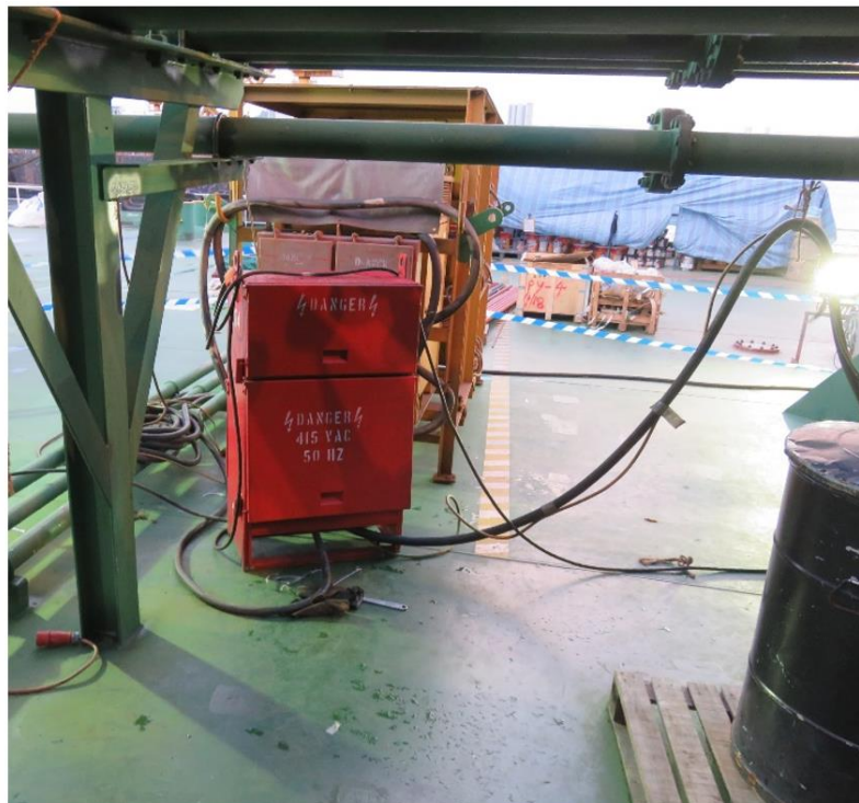
Figure 1: The junction box where electrical cables were being connected.
