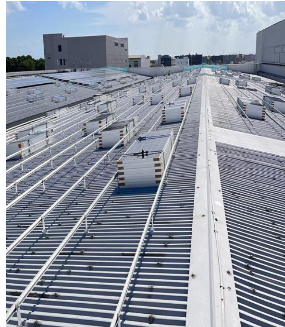
Solar panels secured on roof
