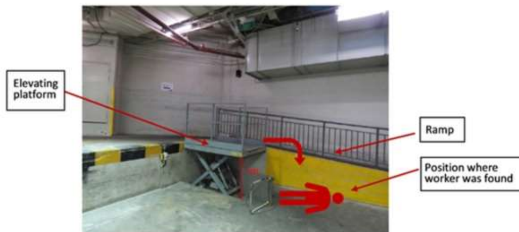
Overview of accident scene.
